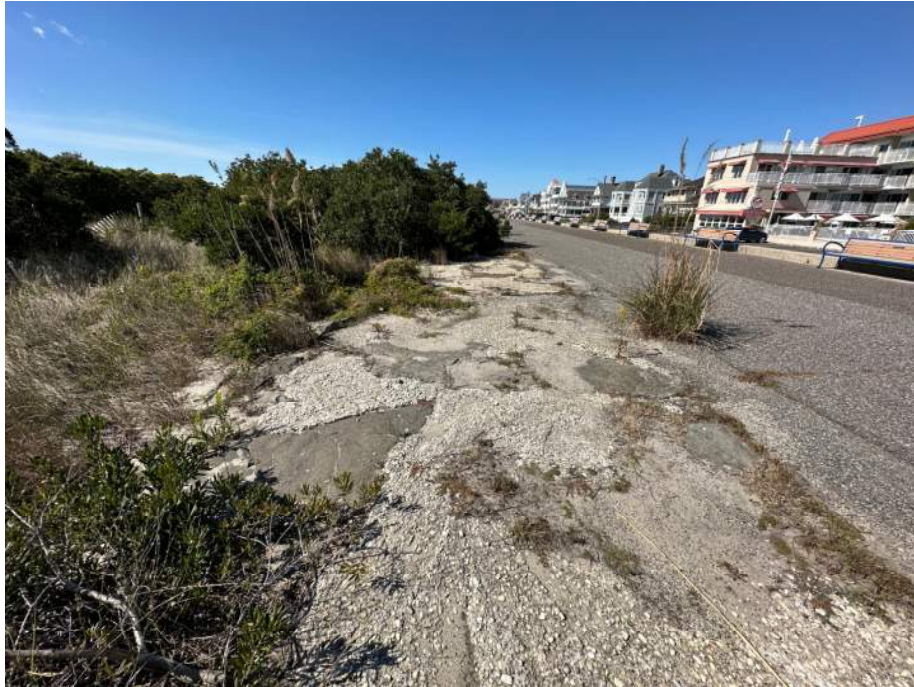
Photo #7 - Existing stone seawall running parralle to promenade.
