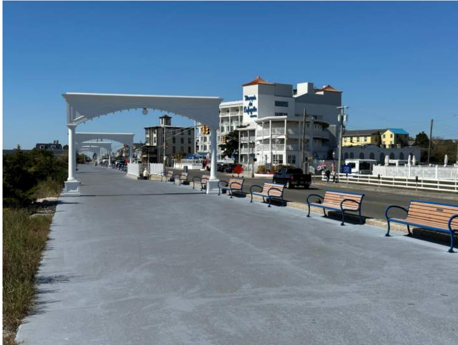
Photo #15 - Area where the promande walking surface has been redone.
